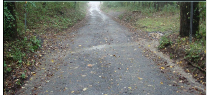
Broad-Based Dip - A small increase in road elevation that directs all road drainage across the road to an outlet.
