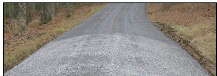
Center Crown – An “A” shaped high point on the road centerline to shed water to both sides of the road.
